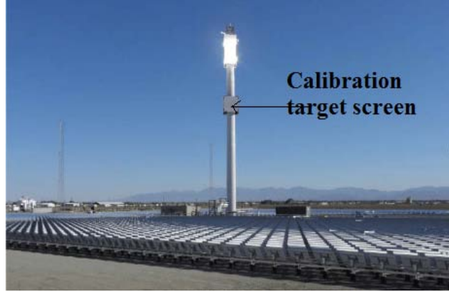
Figure 1.7: Calibration target for open-loop tracking
