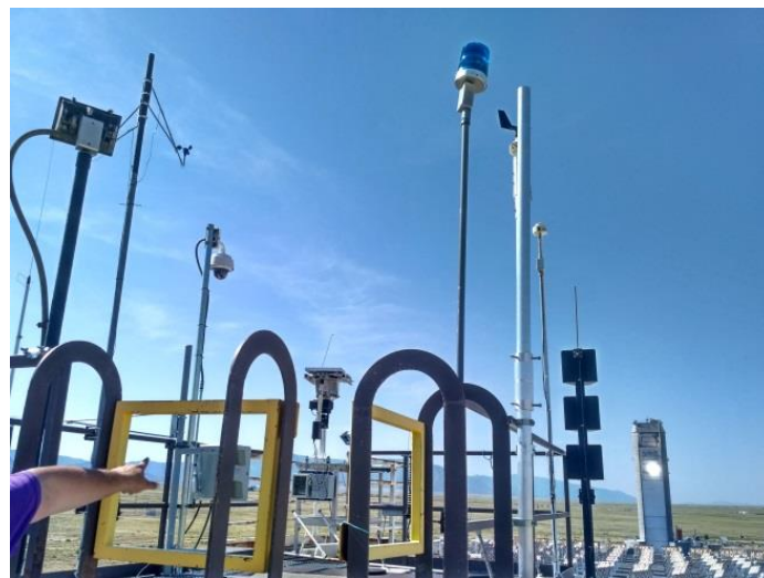
Fig. 6.21: Weather instrumentation mounted on the control room
