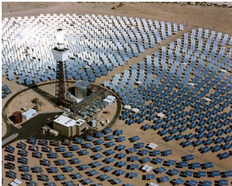
Fig. 2.2: Solar One, Barstow, California [23]
