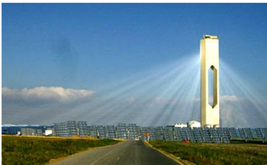
Fig. 2.3: Beams visible due to dust at PS10, Seville, Spain [24]
