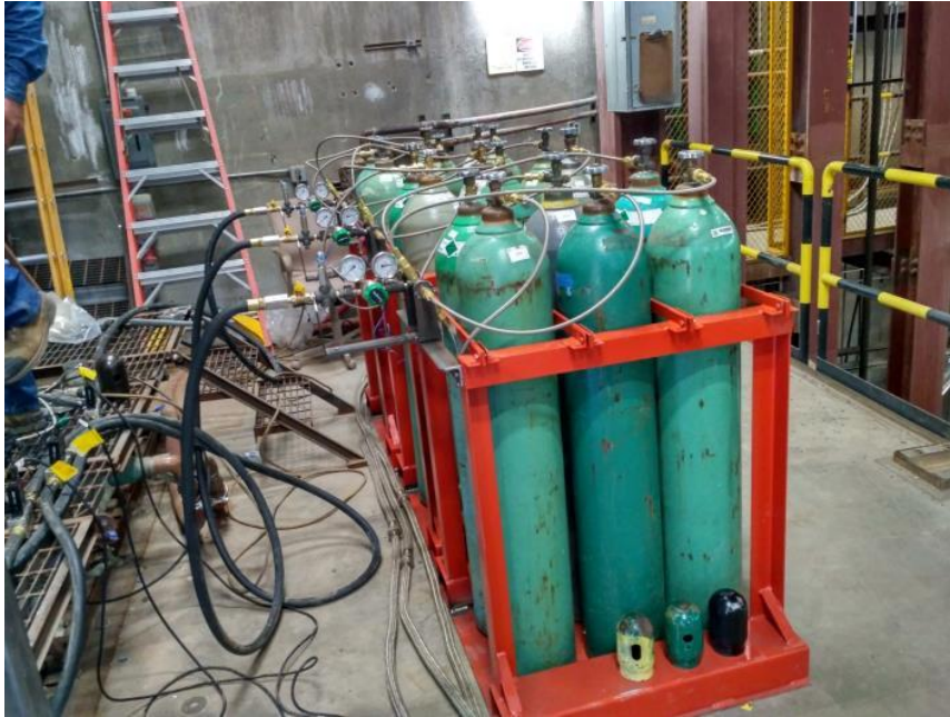
Fig. 6.17: Three stacks of air bottles (6 bottles per stack) located just behind the receiver
