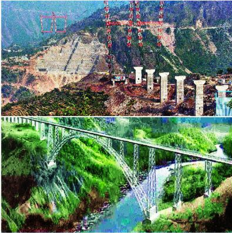
Chenab river bridge, India
