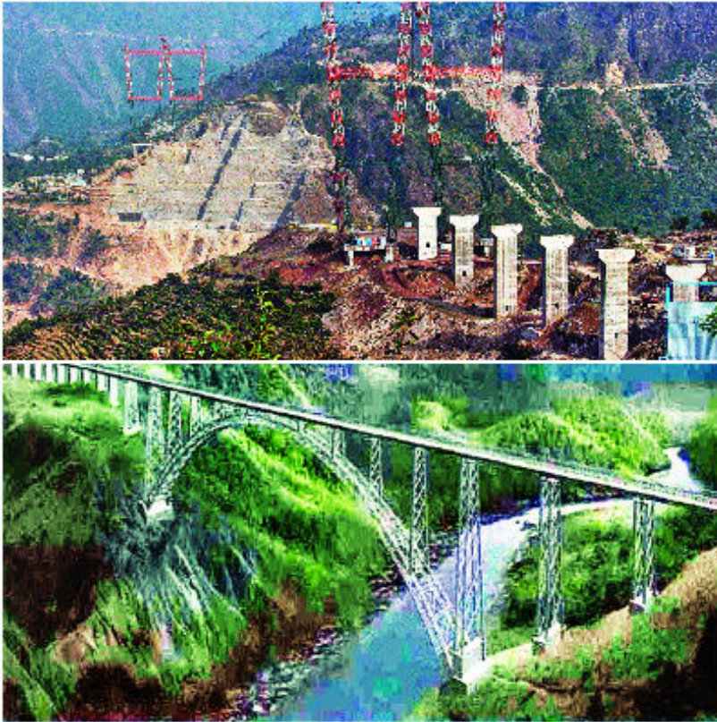
Chenab river bridge, India
